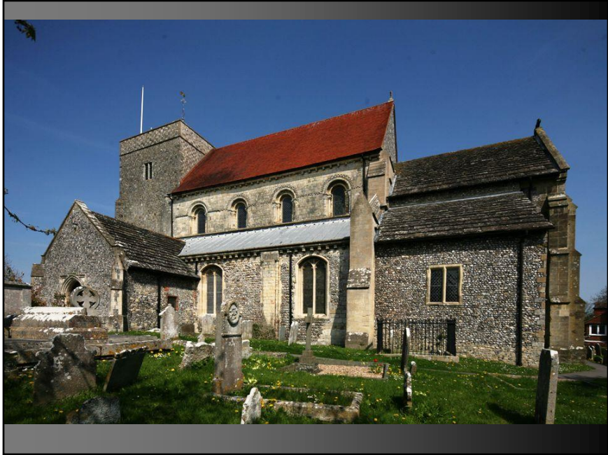
Steyning. South side of Steyning exterior. This weird buttress, very, very unusual.
