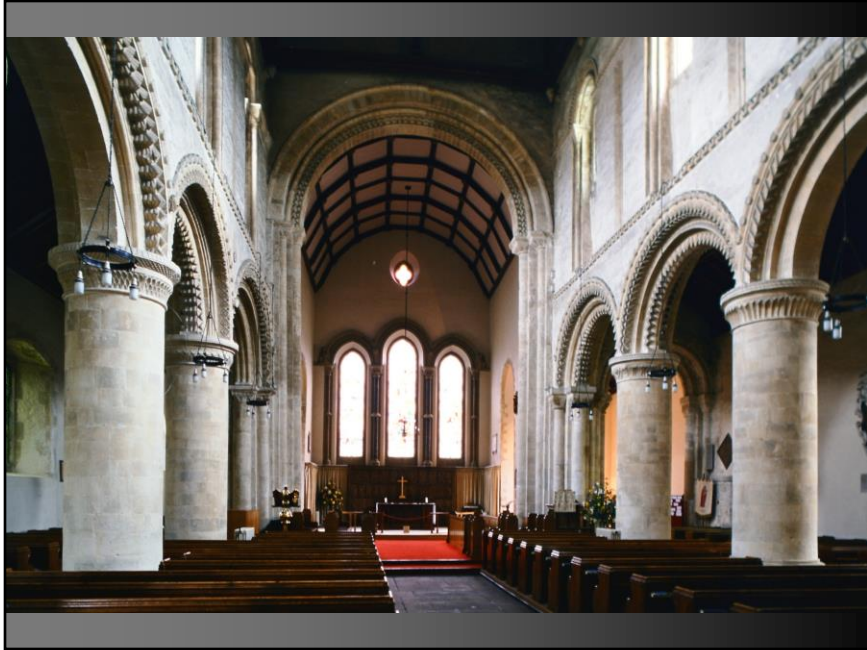
Steyning , view towards the east.
