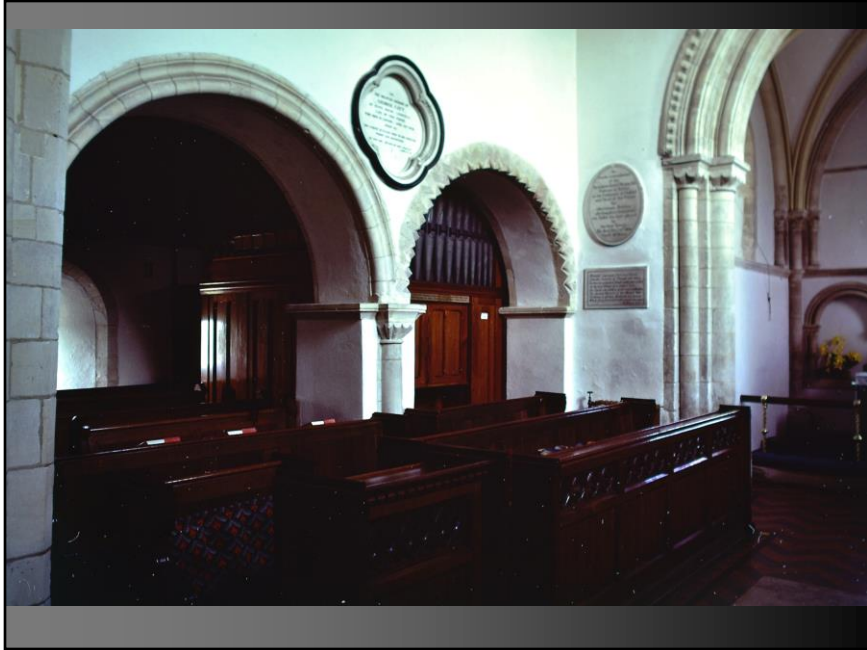
Broadwater – much simpler – moulded arch, chevron arch.
